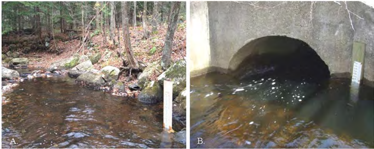
Figure 21. Examples of controls downstream of staff gages include A. riffle and B. culvert.
