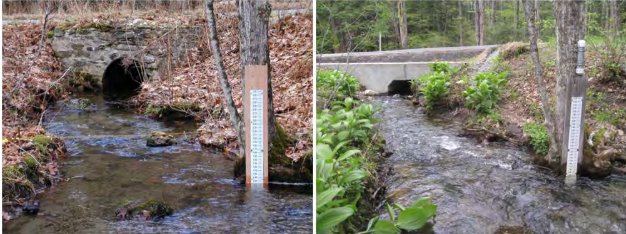
Figure 33. A culvert replacement downstream of a stream gage on Gulf Brook in Pepperell, MA caused enough of a channel change to necessitate a new rating curve.
