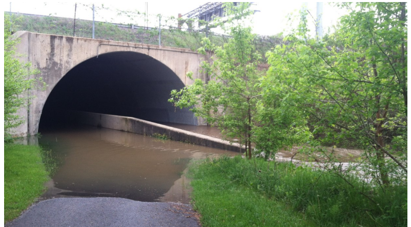
Fig 4. Slab Cabin Run flooding where it is channelized to go under Route 26 in College Township.
