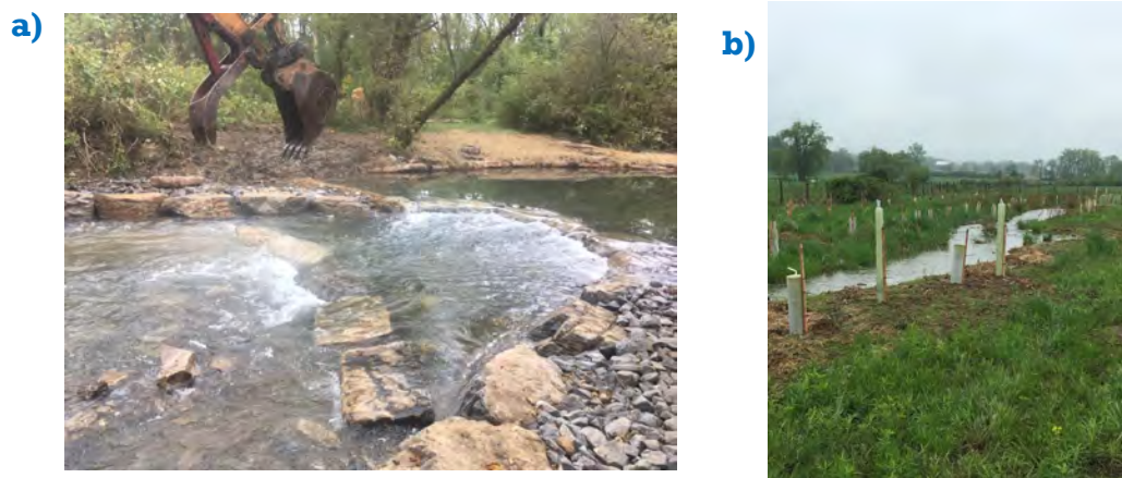
Fig. 26 Examples of stream restoration projects in the Spring Creek Watershed (a) in-stream restoration project in Spring Creek (Spring Creek Chapter of TU) ,(b) riparian buffer restoration on Slab Cabin Run (ClearWater Conservancy)
