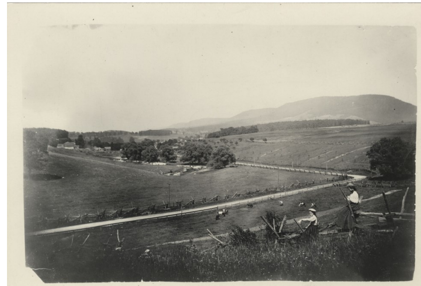
Figure 14. Photograph of Thompson Spring in the Late 1890s showing the current Location of Penn State Wastewater Treatment Plant.
