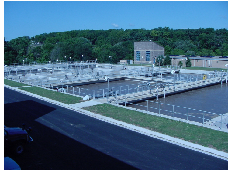
UAJA aeration basins (credit: J. Brown)
