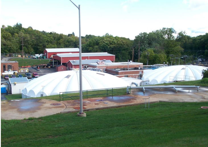
Penn State University Wastewater Treatment Facility (credit: R. Carline)
