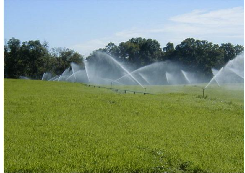
Penn State University Living Filter System spray irrigating treated wastewater on University cropland (credit: John Gaudlip—PSU OPP)
