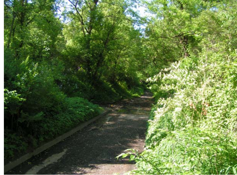
Stormwater Channel in State College Borough (credit: G. Smith)
