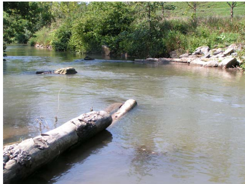
Fish habitat enhancement and stream bank stabilization structure at the PSU Sheep Farm (credit: G. Smith)
