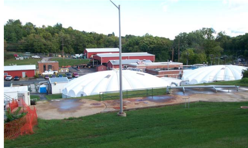
Pennsylvania State University Wastewater Treatment Facility (credit: Bob Carline)
