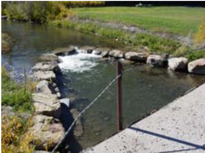
Figure 29. Cross vane structure installed by Dave Rosgen of Wildlands Hydrology, Inc. . Photo: T. Rightnour
