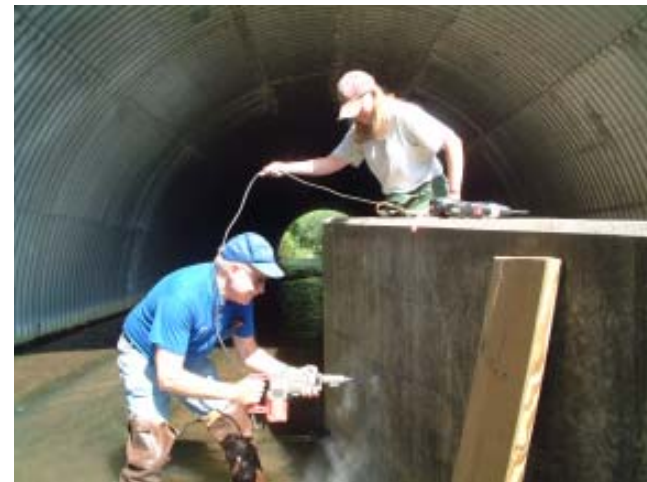
Figure 3. Todd Giddings, water resources committee member, and project staff install monitoring equipment at Slab Cabin Run. Photo: R. Carline
