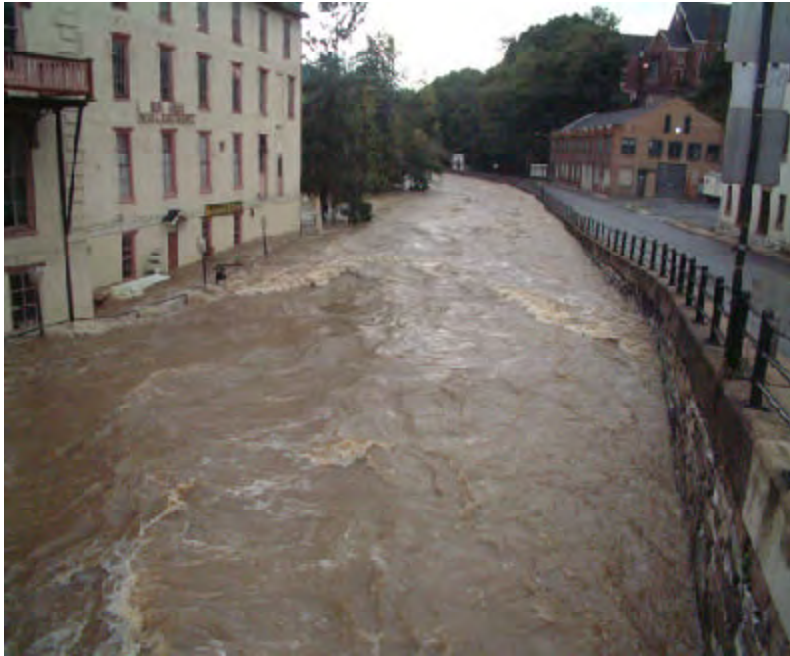
Figure 2. Bush House Hotel, Bellefonte, inundated with flood waters from Hurricane Ivan. Photo: T. Giddings
